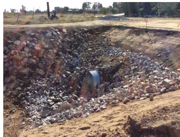
Main canal corrugated metal pipe culvert on east end of crossing (backfilled and riprap).
