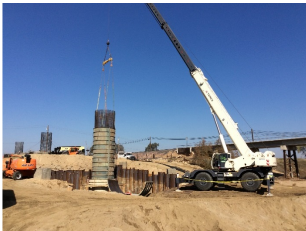
Lifting and installing column formwork at FRV Bent #4.
