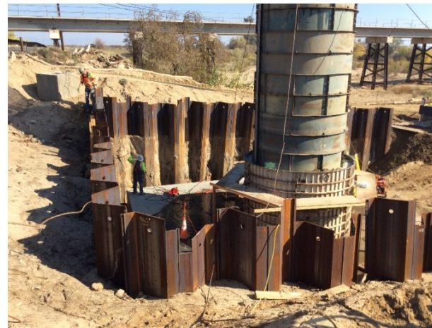
Workers installing column formwork at FRV Bent #4.
