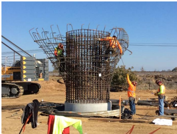
Attaching rebar for column flare at FRV Bent #11.
