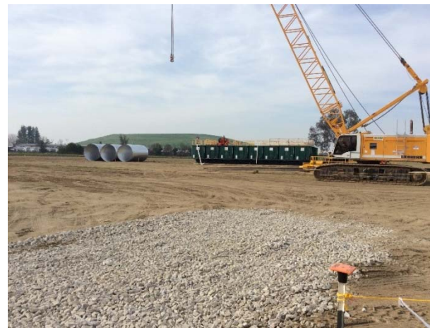
Downtown Fresno Viaduct – construction entrance.
