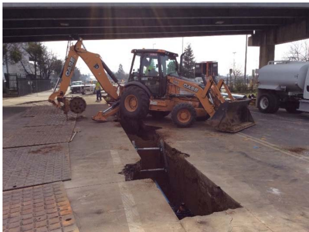
H Street and Tuolumne Street – utility relocation.
