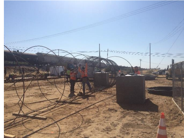
Assembling rebar cage for Column #10 at Fresno River Viaduct.
