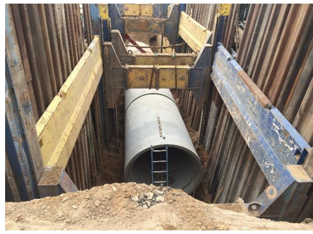
Continuing with 72" storm drain work on F Street.
