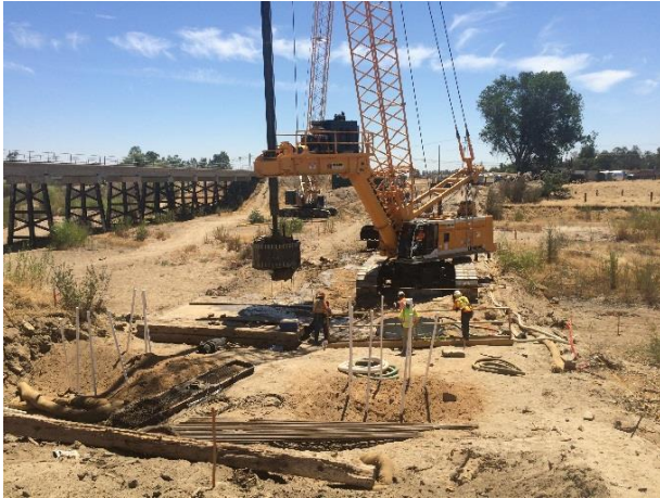
Drilling for CIDH Bent #5 at the Fresno River Viaduct.
