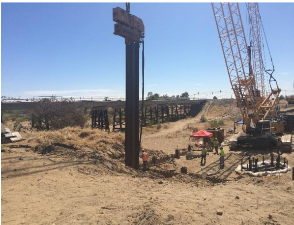
Driving sheet pile for Bent #4 at the Fresno River Viaduct.
